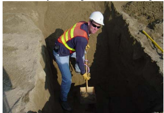
Deep Target Excavation
