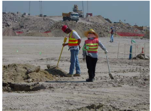
Target Excavation w/ Schonstedt GA-52
